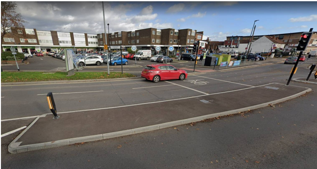
New crossing island in Station Road, approaching Harrow Market
