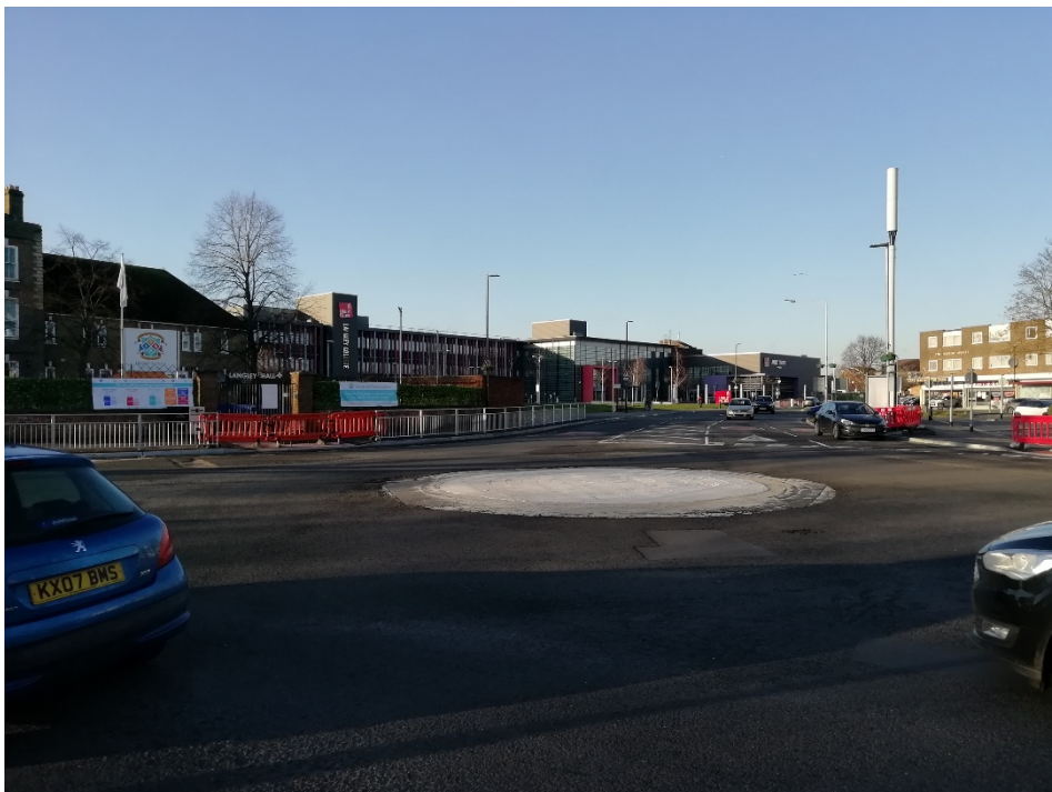
The old roundabout at Harrow Market, shortly before being replaced
